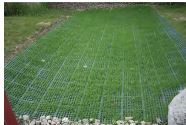
The RevetMax ShoreMax Transition Mat help vegetation growth through voids in the mat.
