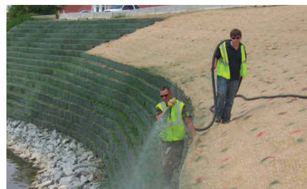
The North American Green HydraMax System can be installed three times faster than erosion control blankets with 1/3 of the labor costs.
