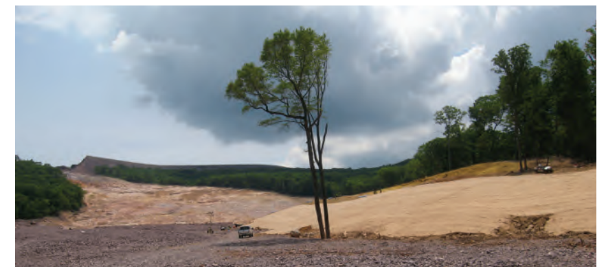
North American Green Erosion Control Systems are recognized as EPA Best Management Practices (BMPs) that help you comply with regulations and protect valuable resources.
